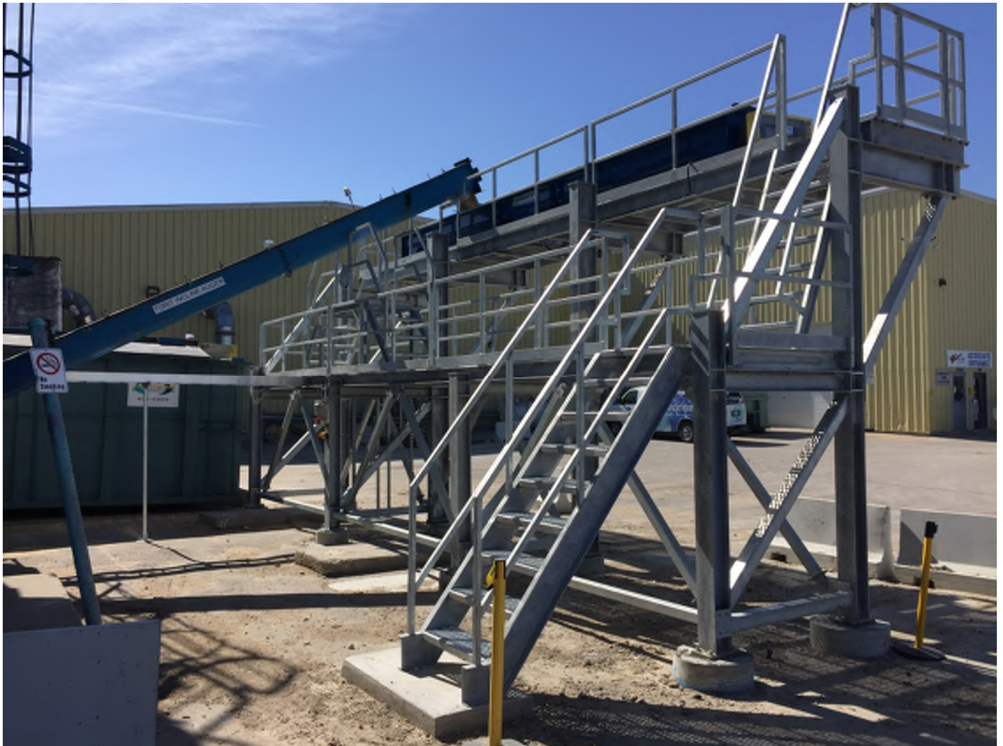
Conveyor access platform
