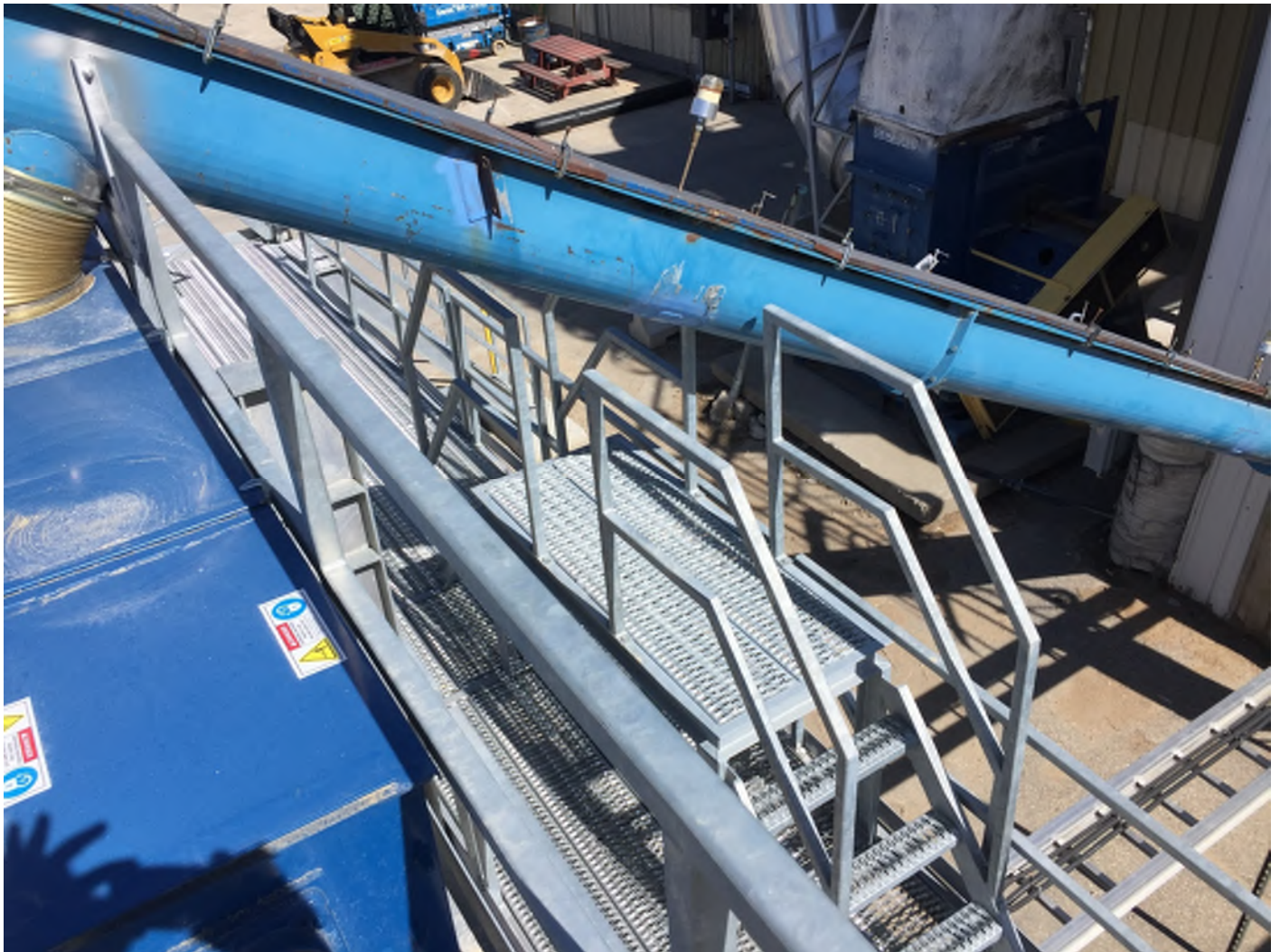
Conveyor access platform
